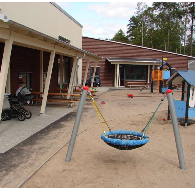
Energy efficient preschool with passive building technology, Stadsskogen Alingsås Photo: Municipality of Alingsås
